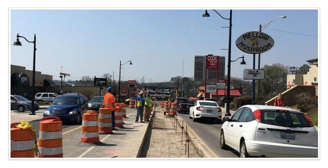
Mid-block left turns have been prevented so far by temporary barriers. The new medians will be between 3 feet and 13 feet wide, depending on turn lanes and Knoxville Area Transit bus infrastructure. Even though the number of traffic lanes on Cumberland has been reduced, the design is expected to reduce fender benders and improve traffic flow by eliminating blockages created by vehicles turning left across incoming traffic in the middle of the block.
