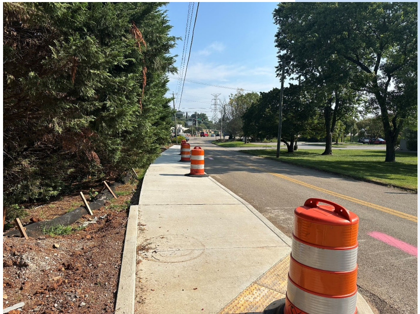
Ongoing Construction at Golfclub Road August 2023
