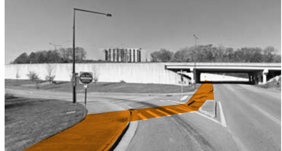
Connection to James White Greenway
