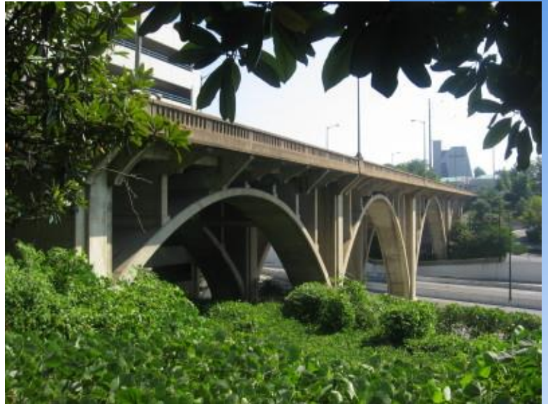
Hill Avenue Viaduct
