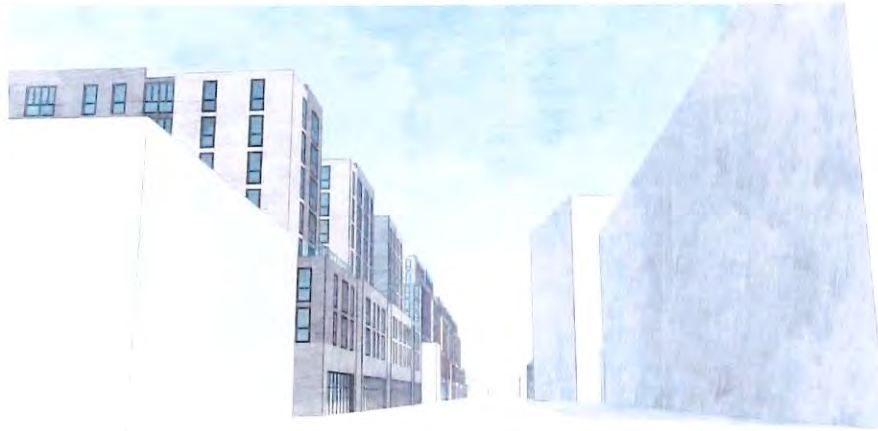
VIEW EAST DOWN CUMBERLAND
