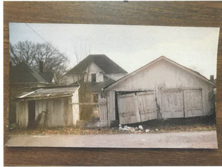
PREVIOUS OUTBUILDINGS, VIEW FROM ALLEY (photo circa 2006)
